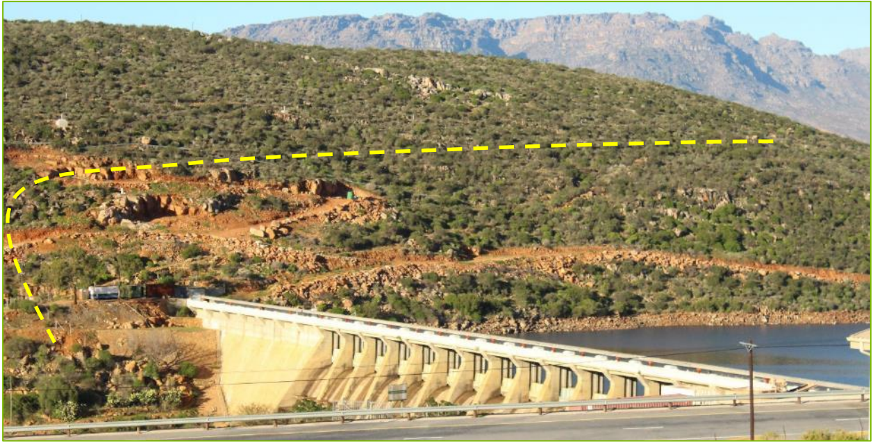
Figure 6: Rising Main 2 Route - view from left bank of Clanwilliam Dam
